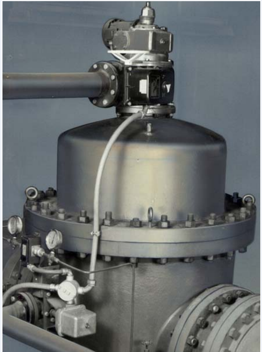
A Model LDP installed in a piping system
